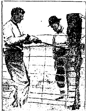
Attaching the Wire After It Has Been Stretched.
